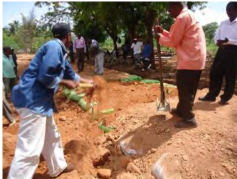
Demonstration of the works by community Raised-up Toilet
