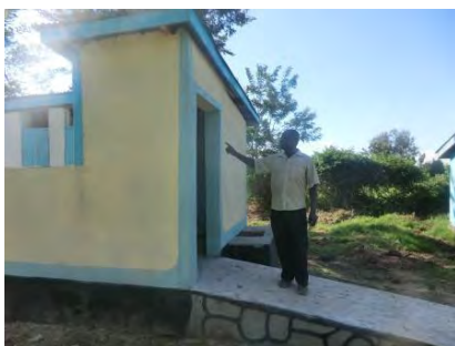
Raised toilet constructed at Nyora Primary School located in flood prone areas, LOGUMI WRUA influenced the design change from ground level design to raised above flood depth design
