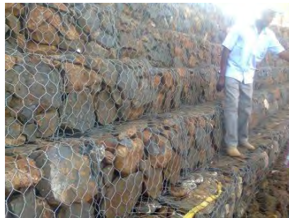
Excursion visit to isiolo river basin where WRUA members observed riverbank protection in flood prone areas
