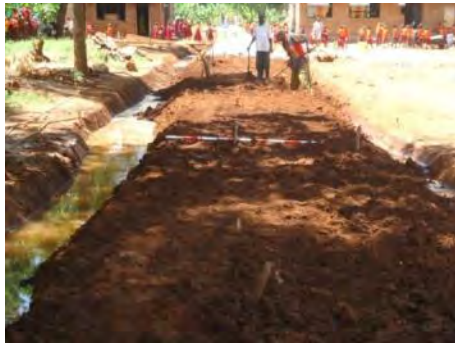
Preparation of the road surface and drainage
