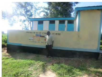
Raised toilet constructed at Nyora Primary School located in flood prone areas, LOGUMI WRUA influenced the design change from ground level design to raised above flood depth design
