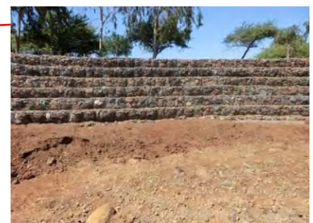
After bank protection using gabion box
