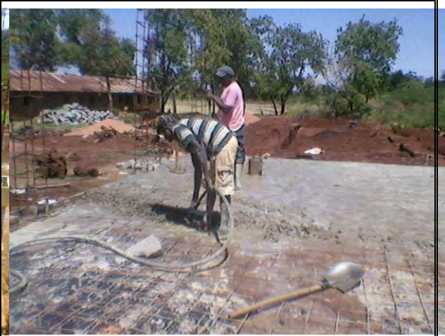
Date: 20-01-2014 Description: Concreting the floor slab
