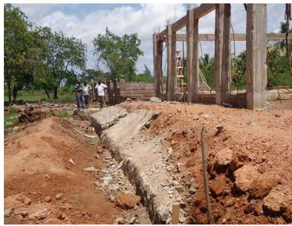
Date: 24-02-2014 Description: Completion of Structural frame of columns and beams
