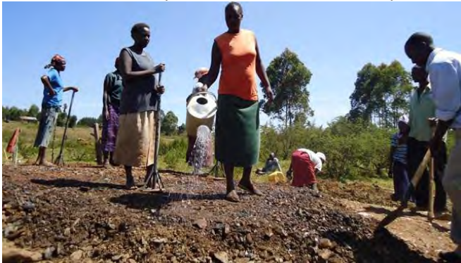
If the soil is too dry, water it to facilitate compaction
