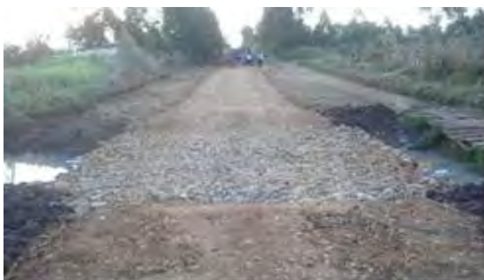
Make a firm drift foundation made of hardcore
