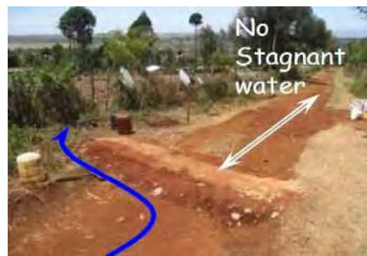
Check that the gradient slopes for water flow
