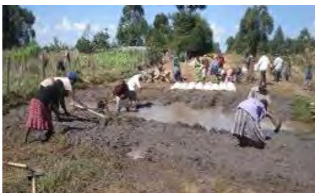
Remove unwanted soft material
