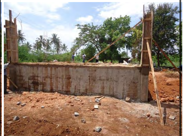
Date: 22-01-2014 Description: Concrete Works for the Columns
