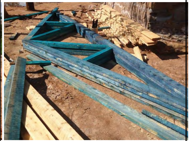
Date: 28-02-2014 Description: Fabrication of roof trusses
