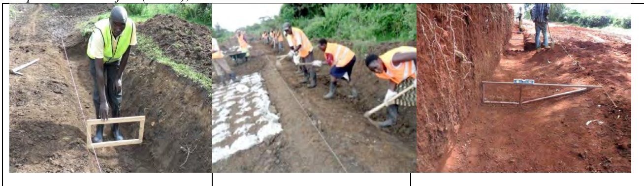
Control ditch excavation width using ‘ditch template’
