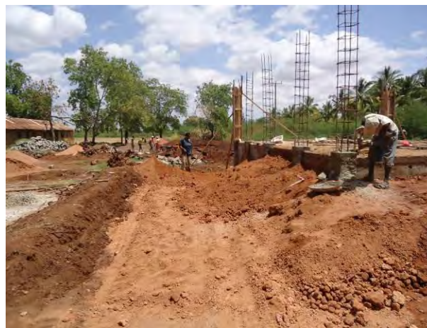
Date: 22-01-2014 Description: Reinforcement for the Columns
