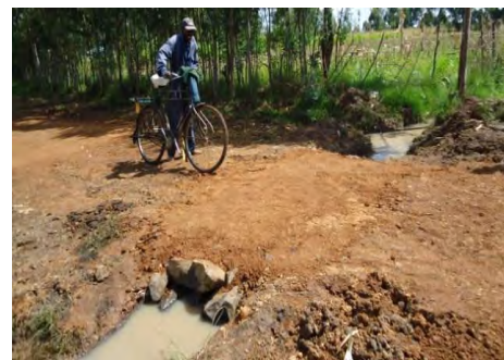
Do-nou bags which are filled with in-situ soil
