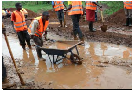
If there is mud, remove and dispose off
