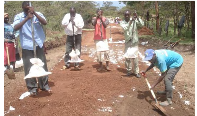
Check camber formation to ensure water is drained away from the carriageway
