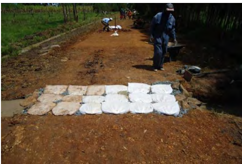
Lay Do-nou bags appropriately and compact
