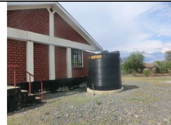
Description : Well-maintained water tank that is used for drinking in the village. CFMO charges Kshs. 2/- per 20Lts gallon
