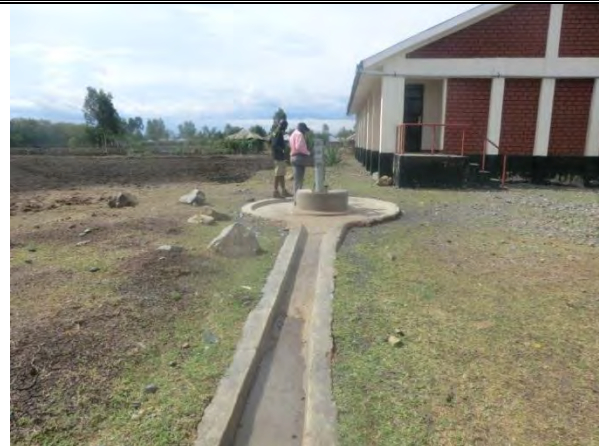
Description : CFMO at Kanyango has managed to install a 60M deep borehole with a handpump at EVC
