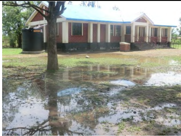
Description : Raised Evacuation centre above flood depth
