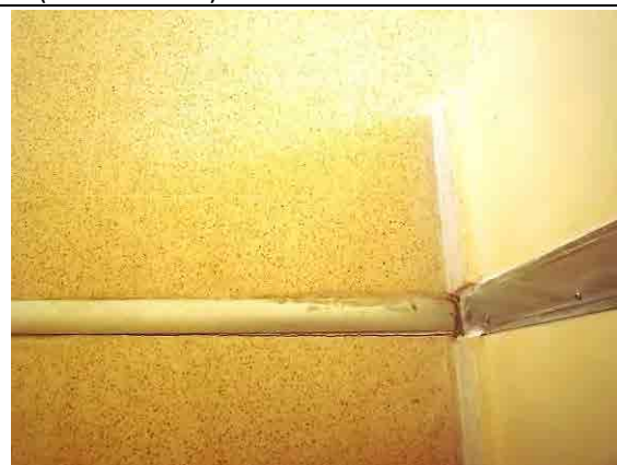
Expansion joint having cracks on the floor (28 Nov. 2012)
