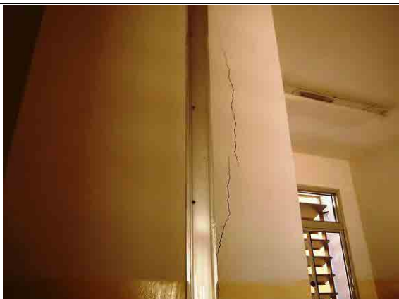
Expansion joint having cracks on the wall (28 Nov. 2012)
