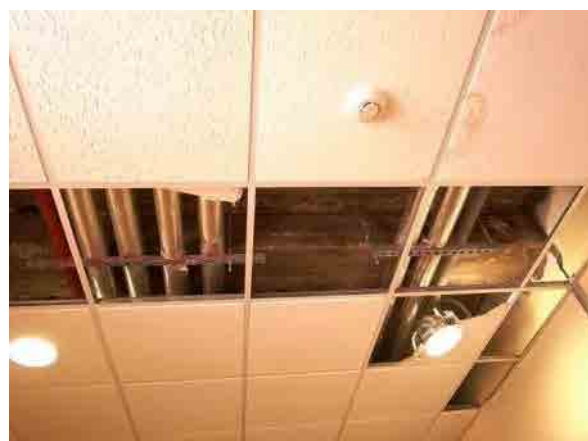
Some parts of ceiling boards had been fallen.
