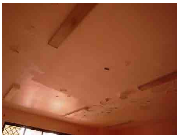
Water leakage could be confirmed.
