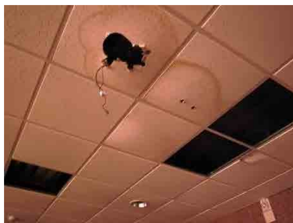
Due to water leakage, some lighting had been broken.
