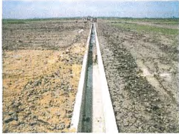
[Completion of Construction] (Thomney Model site)
