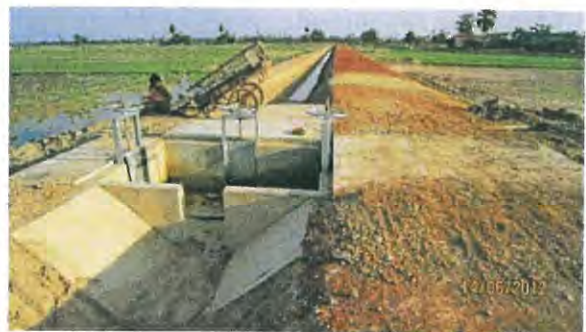
[Completion of Construction] (Roleang Chrey Model site)
