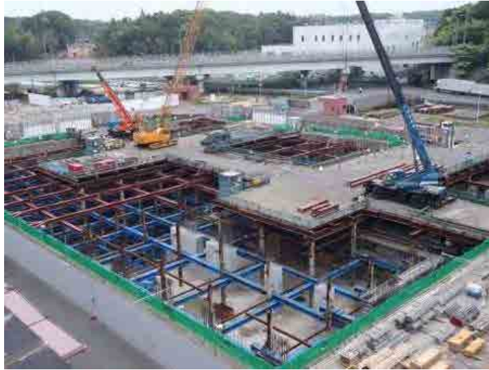
Figure 3.16 Example of Temporary Earth Retaining Wall
