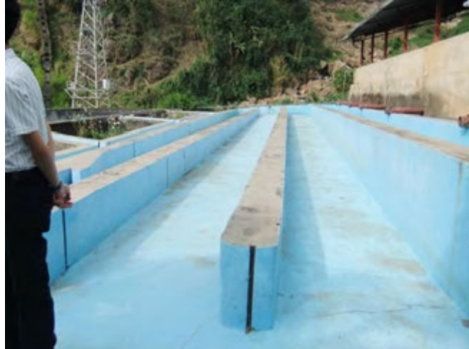
Photograph 4-8: Excessively wide water channel (Rwanda)
