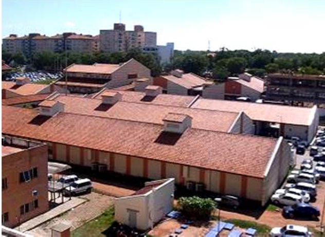
Building constructed under the Project
