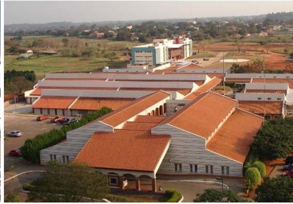
CMI (front) and Outpatient Building for Pediatrics Department (rear)
