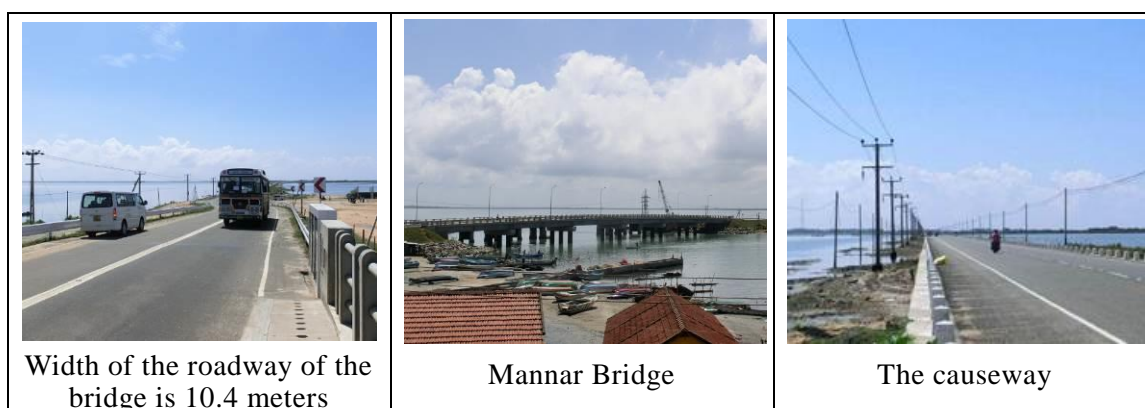
The new Mannar Bridge and the improved causeway
