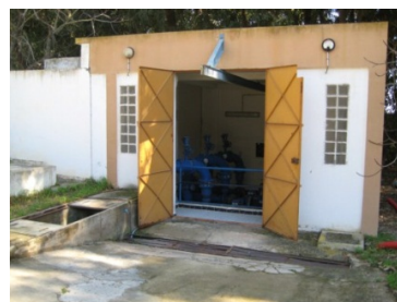
Takabrote Pumping Station
