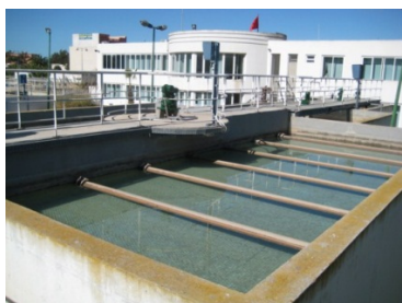
Safi Water Purification Plant
