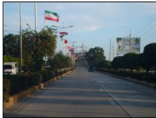
Second Mactan Bridge (Mandaue Side)
