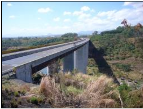
Gumain River Bridge
