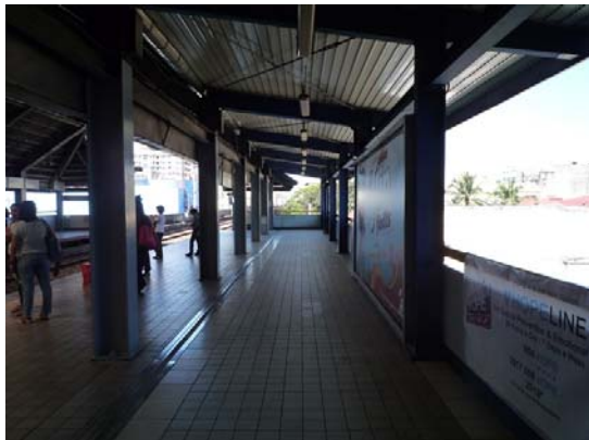
Expansion of Platform (EDSA station)
