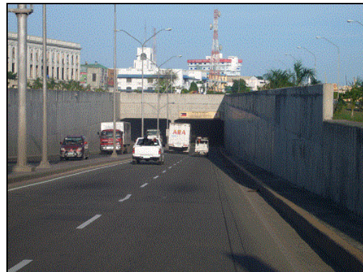
Coastal Road (Tunnel section)
