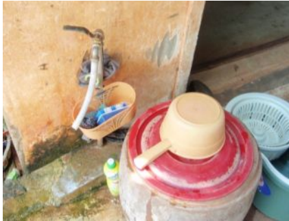
Water faucet at a beneficiary household. Prior to the project, the family used a dug well. Now tap water is the main source of water for cooking, drinking, washing, etc., and the amount of water used has doubled from before the introduction of tap water.
