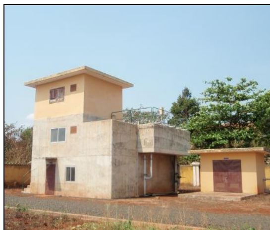
Water Supply Facility at Nhon Hoa, Gia Lai Province
