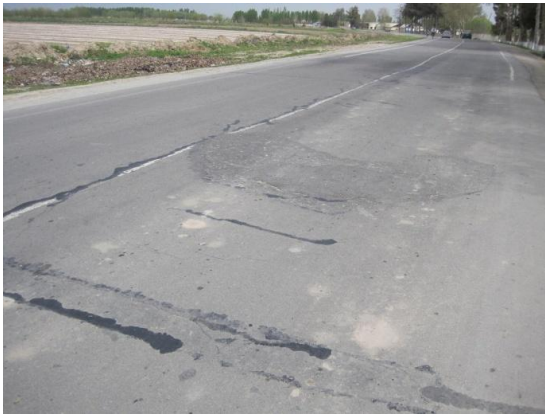
Photo 4: Road surface repaired after damages (Phase I section: surfaces are undulating and the median line is winding.)
