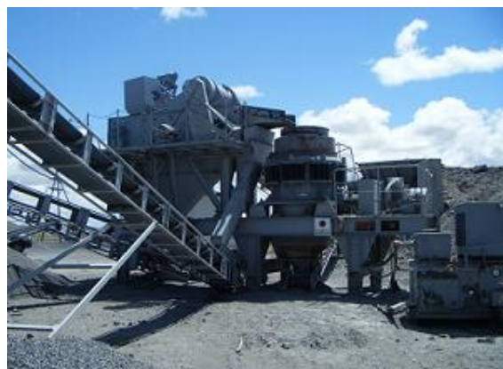
(Photo) Procured equipment: Crasher plant
