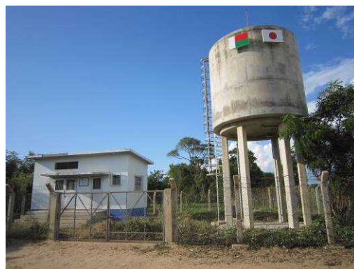
Public fountain type water supply facility
