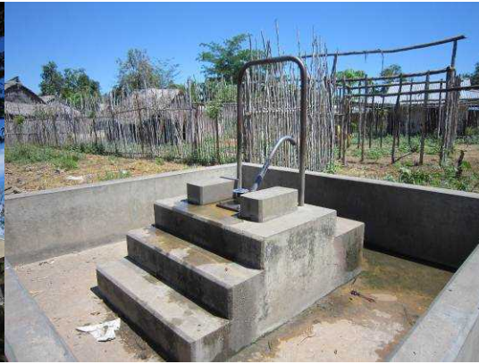
Photo 2: Foot pump type Water supply facility
