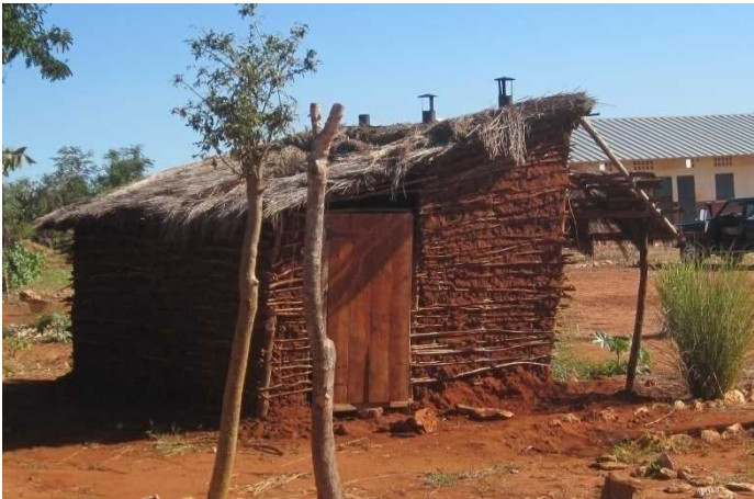
Classroom with Clay Wall Constructed by the Community
