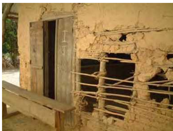
Classroom with Clay Wall Constructed by the Community
