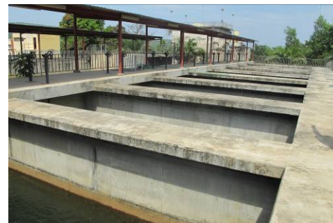
3 rd Water Treatment Plant in Yessoulou (Rapid filter)
