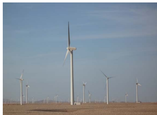
Wind Power Plant Constructed by the Project
