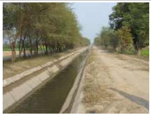
Lining of distributary
