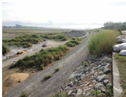
Earth dike in San Nicolas
