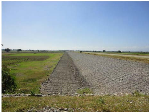
Closure Dike (taken from side)
