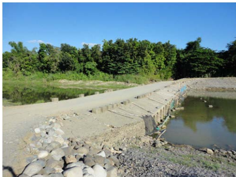
Grade Control Structure
