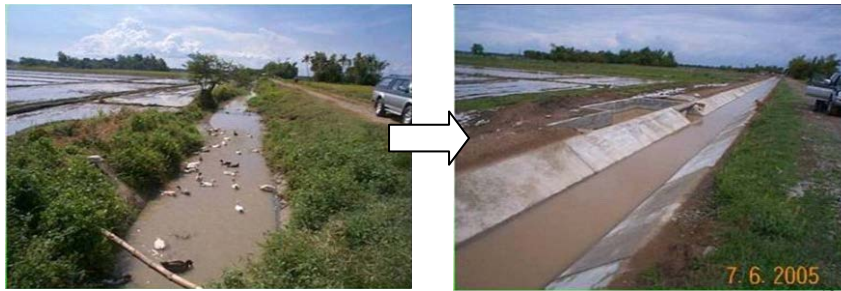
Figure 3: Before and After the Rehabilitation of Secondary Canal 12
