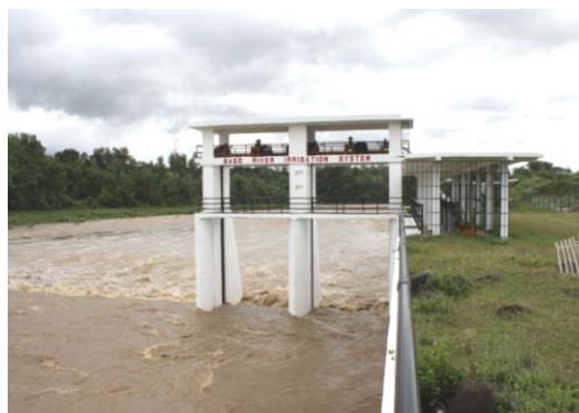
Figure 14: Rehabilitated Weir and Bago River
