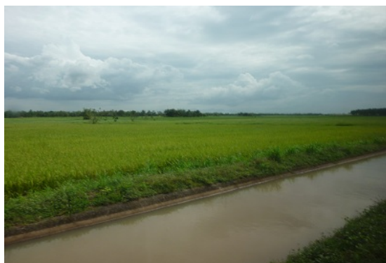
Figure 13: Rehabilitated Main Canal
