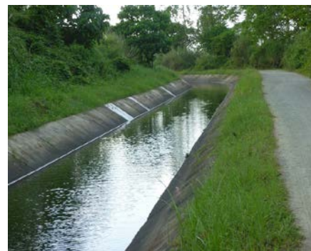
Constructed Main Canal
