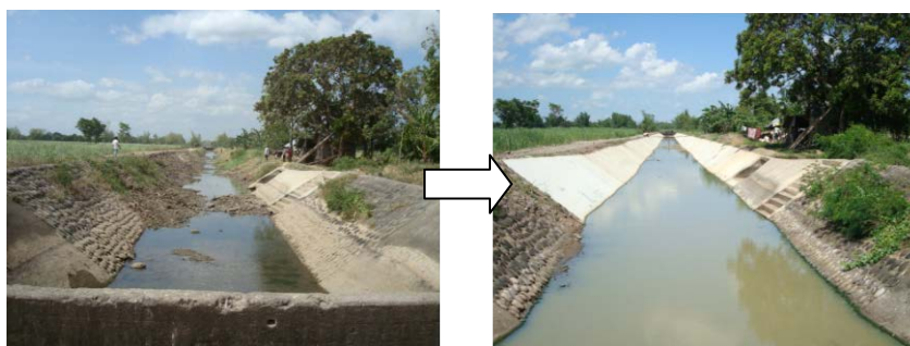
Figure 2: Before and After the Rehabilitation of Main Canal
