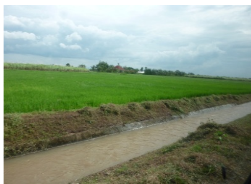
Rehabilitated Secondary Canal
