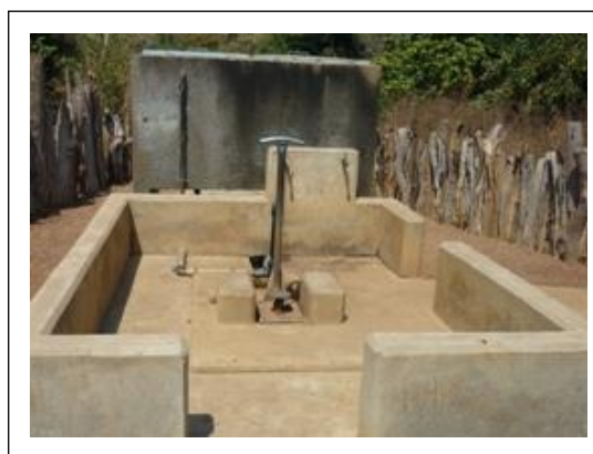
Foot-pump water facility with iron remover provided by the project
