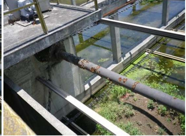
Primary treatment facility not available for operation (Alegria WWTP)
