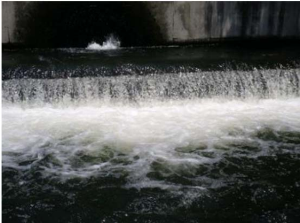
Treated Water Before Discharge (Alegria WWTP)
