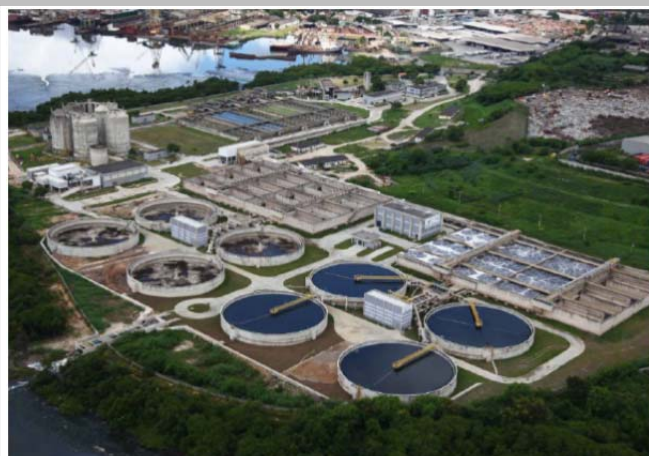
Alegria Waste Water Treatment Plant
