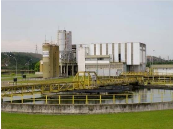
Primary Treatment Facility (Sarapui WWTP)
