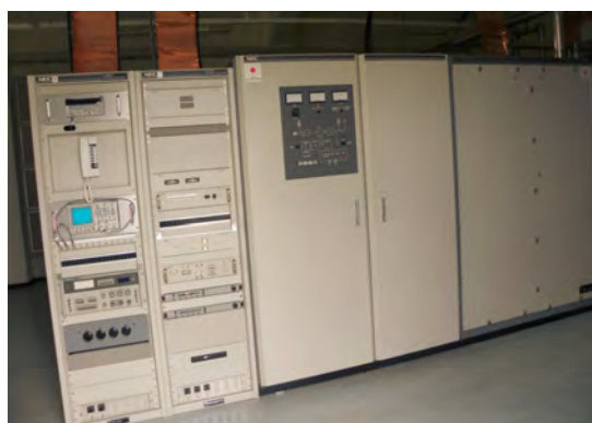
Figure 14: Transmitting Equipment procured for Kyeriba MW Transmitting Stations
