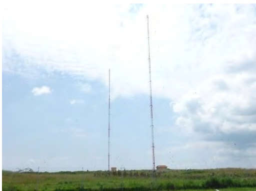
Figure 11: Antenna System at Mawagga Transmitting Station
