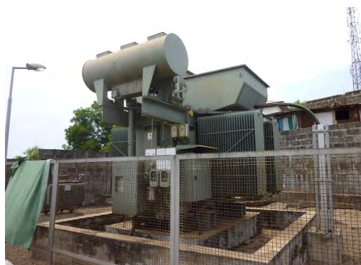
Figure 15: Procured Power Distribution Transformer (Inside the Regent Substation)
