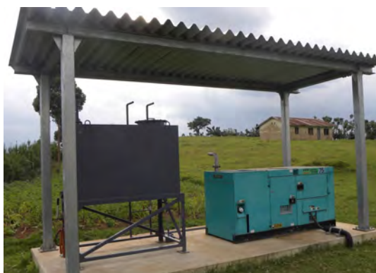
Figure 13: Emergency Generator for Kyeriba MW Transmitting Station (The one on the left is a diesel fuel storage tank.)
