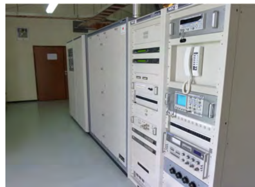
Figure 12: Transmitting Equipment inside Mawagga Transmitting Station
