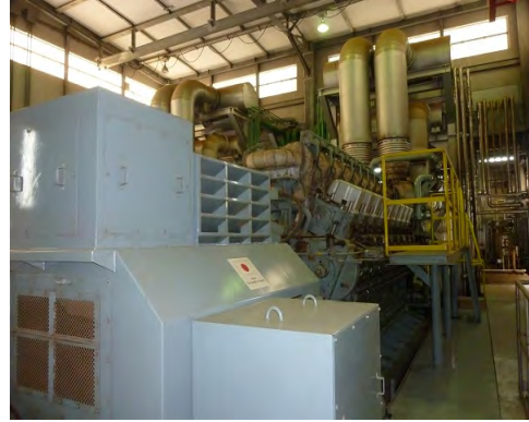
Power Generating Unit Procured by the Project (Kingtom Power Station)
