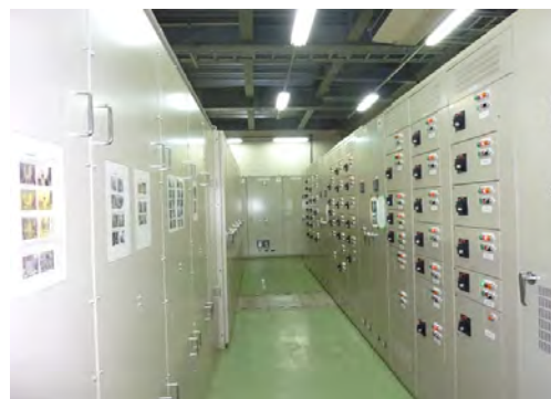
Figure 13: Power Distribution Unit Control Room (Inside the Kingtom Power Station)
