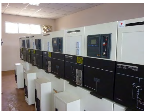
Figure 14: Power Distribution Control Room (Inside the Regent Substation)
