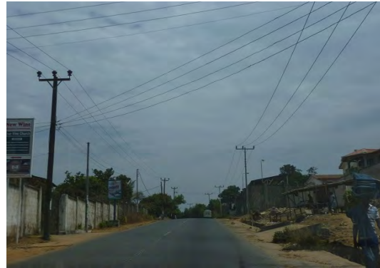
Figure 4: Distribution Line Between Wilberforce and Regent (Left: 11 kV Distribution Line, Right: 33 kV Distribution Line)
