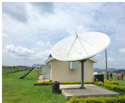
Mawagga MW Radio Transmitting Station
