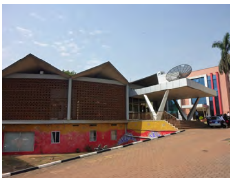
Figure 2: UBC Kampala Broadcast House
