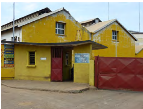
Figure 12: The Exterior of the Kingtom Power Station
