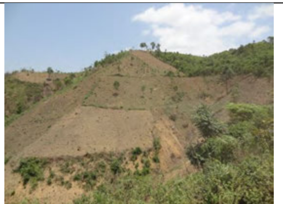
Slope above Luong Luong Dam (Muong Phang Commune)
