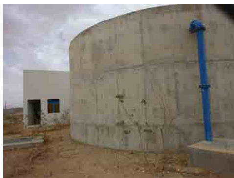
Constructed Reservoir (May-Dima)
