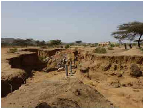
Figure 9: Interrupted Water Transmission Pipe Due to Soil Erosion 42 (Dekemhare)
