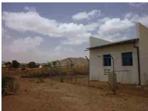
Figure 1: Pumping Facilities (May-Dima)
