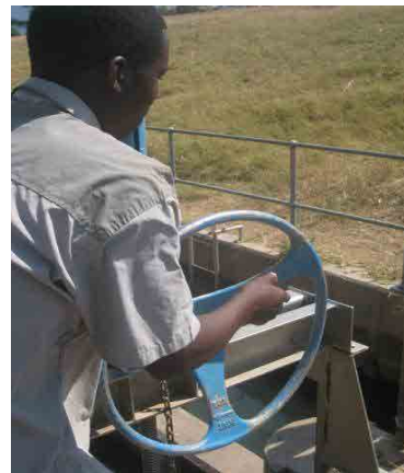
Picture 6 : Water guard controlling the gate of settling basin
