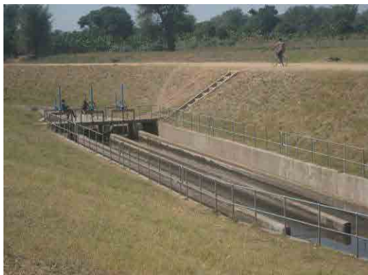
Picture 3 : Newly Constructed Settling Basin
