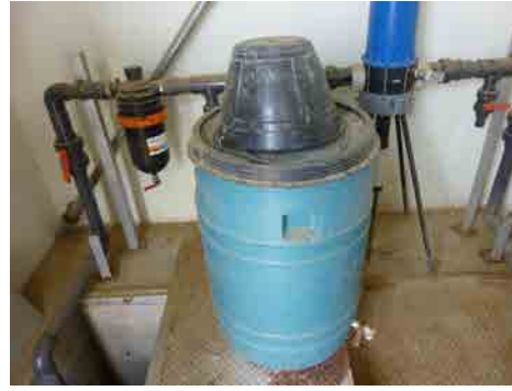
Figure 8: Chlorine Injector
