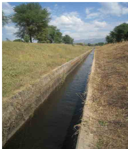
Picture 1: Relocated main canal
