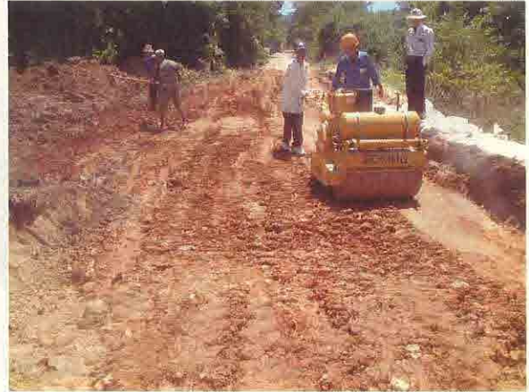
Repair construction road on Pol pot 63
