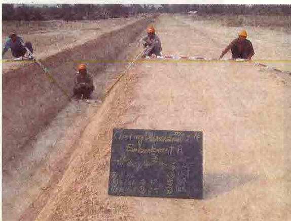
Control of finished work quality
