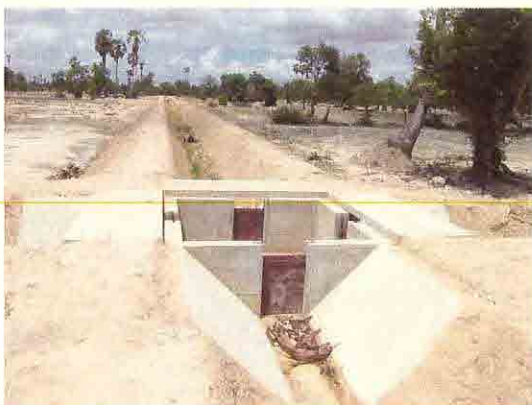
Canal T340, Length=790m Bed width=0.5m Embankment H=0.85m
