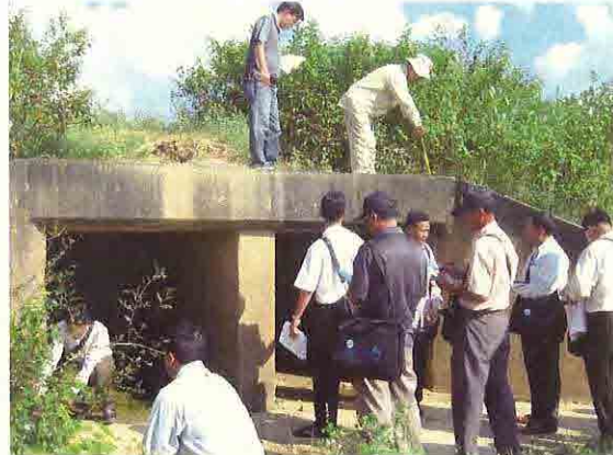
Observation of box culvert by participants during training
