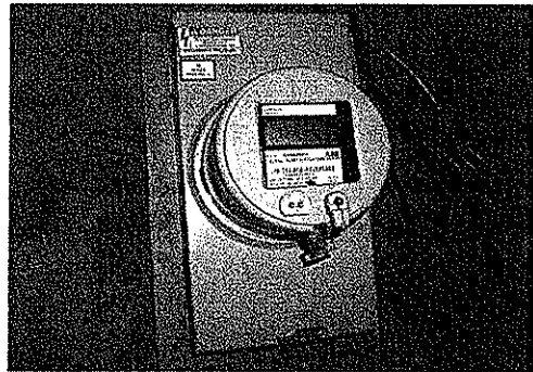
Electric Power Meter
