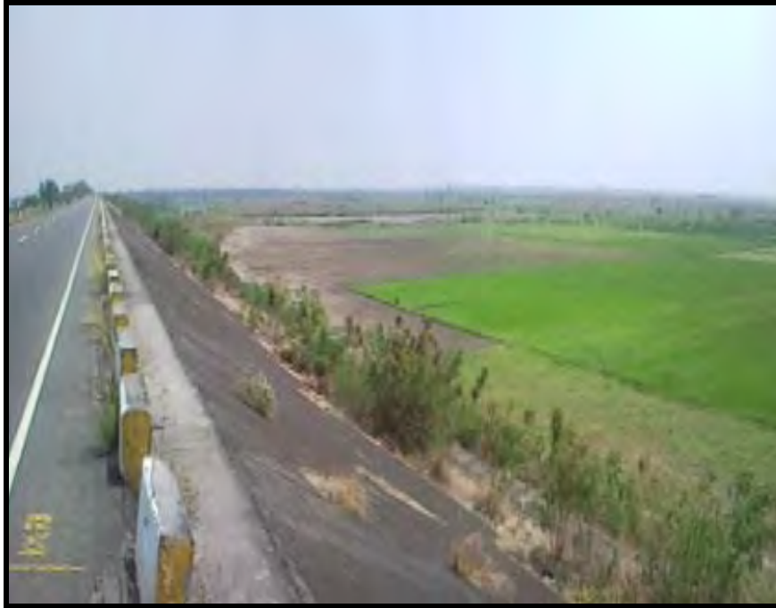
Plate 1 Portion of Sta. Rita dike used as alternate road blocking direct access to the Pasig-Potrero River
