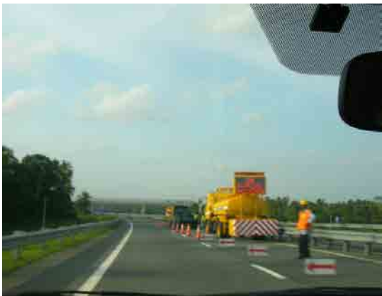
Maintenance work in through lane of Expressway
