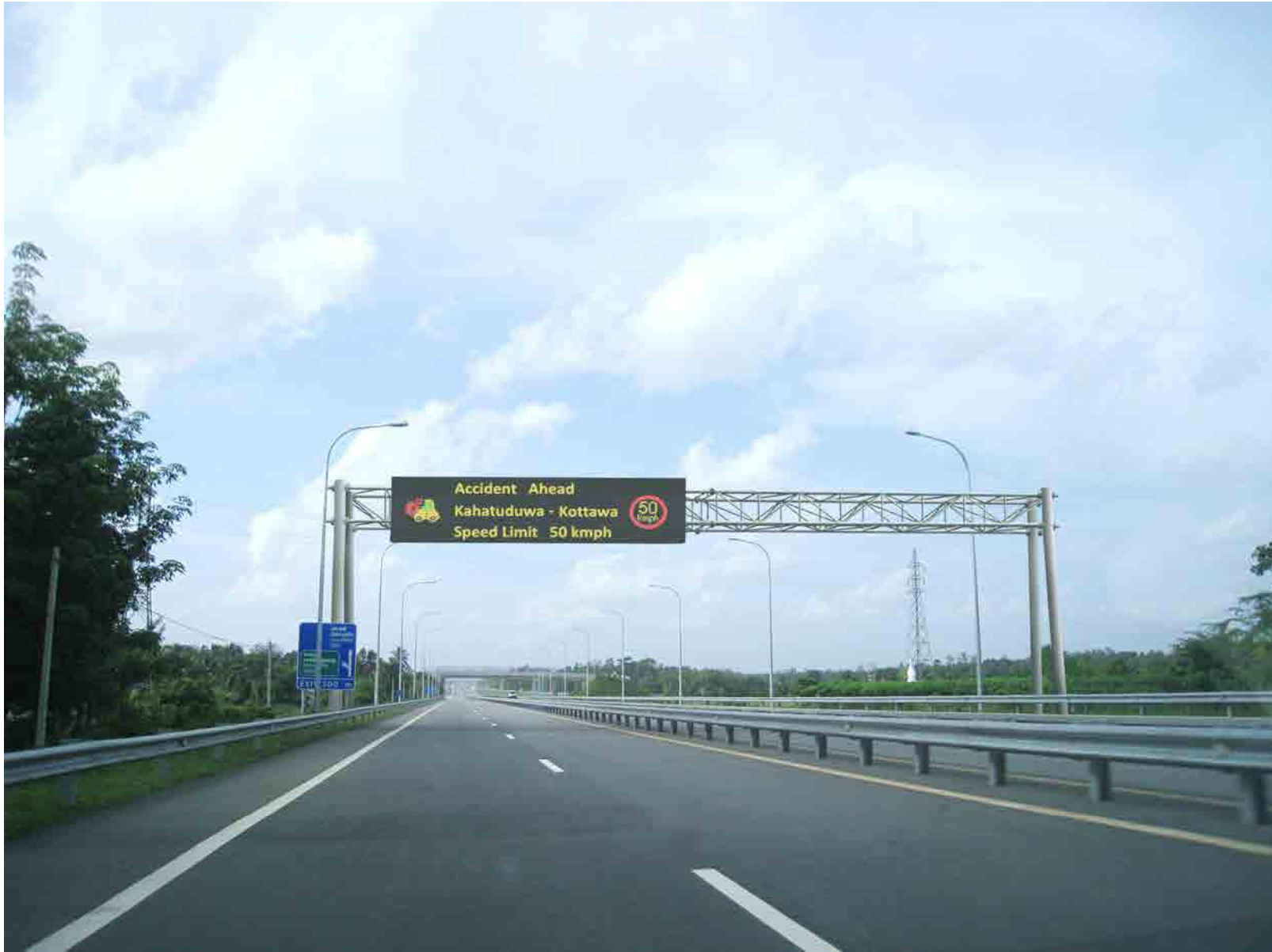
PERSPECTIVE / SOUTHERN EXPRESSWAY Variable Message Sign Board
