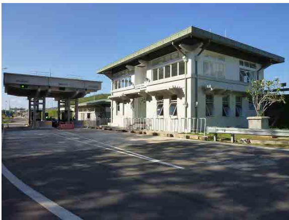
Welipenna Toll Office
