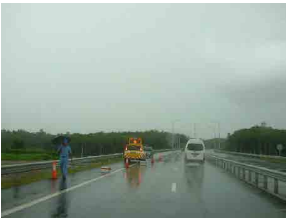
Recovery work for Spine out vehicle due to rain fall
