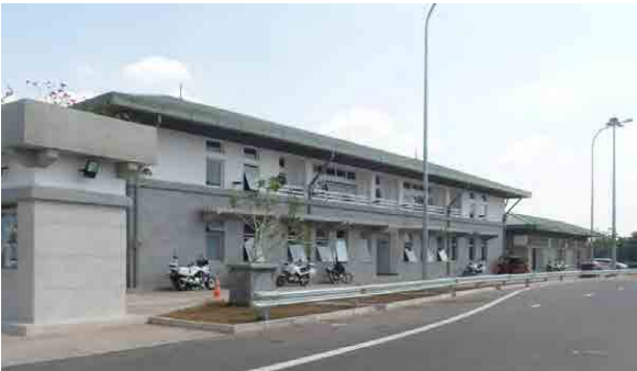
Gelanigama Traffic Control Center
