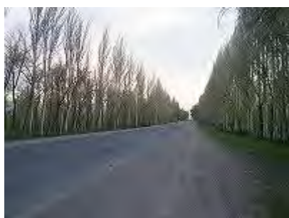
2013-04-28 Issyk-Kul, Tup District Condition of Road maitenance
