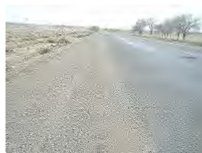
2013-04-25 Issyk-Kul Condition of Road
