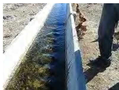
2013-02-16 Tong District Water supply
