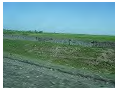
2013-05-10 Chuy Province Water Channel
