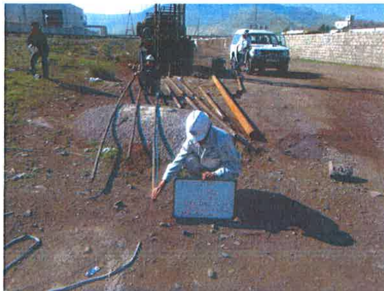
Photo-4 Certification the length of S.P.T No.4 L=19.0m
