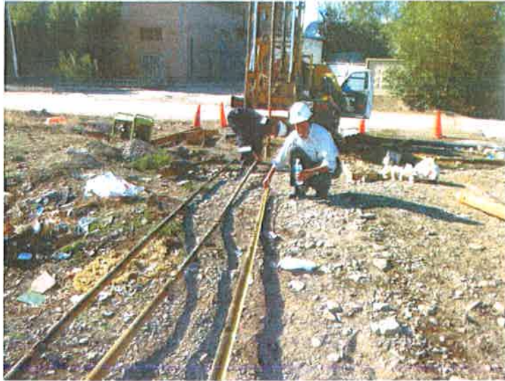
Photo-1 Certification the length of S.P.T No.1 L=19.0m
