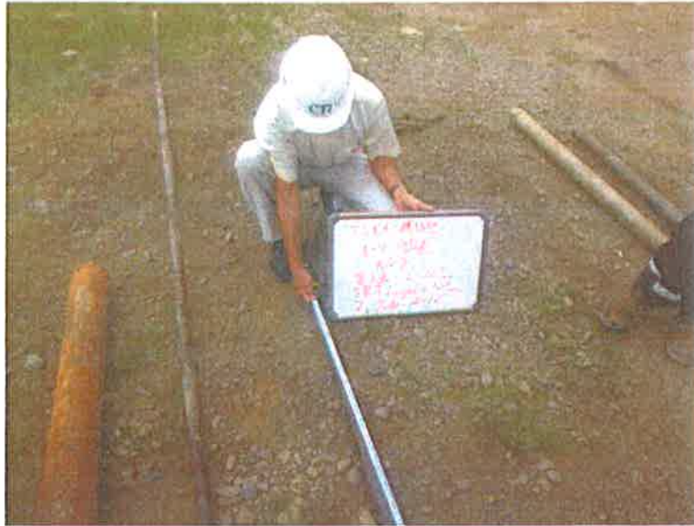
Photo-7 Certification the length of S.P.T No.7 L=12.0m
