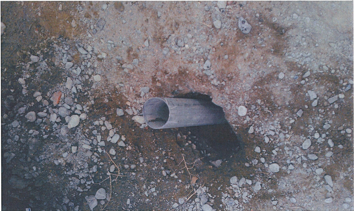
Monitoring Borehole for Further Research
