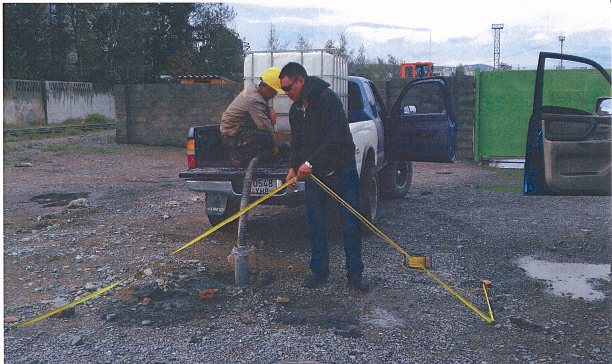
In-situ Permeability Testing
