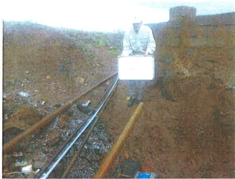
Photo-3 Certification the length of S.P.T No.3 L=12.0m
