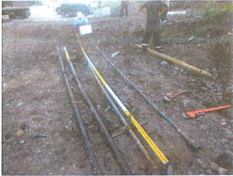
Photo-11 Certification the length of S.P.T No.11 L=13.0m
