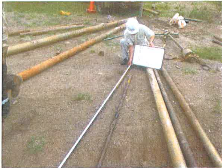
Photo-5 Certification the length of S.P.T No.5 L=16.0m
