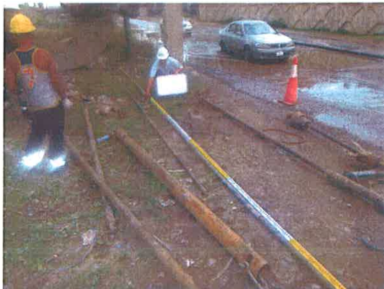
Photo-10 Certification the length of S.P.T No.10 L=14.0m
