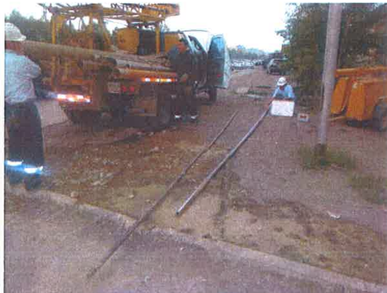
Photo-8 Certification the length of S.P.T No.8 L=14.0m
