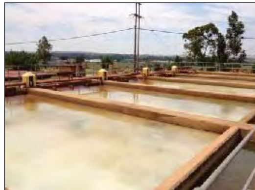
Bronkhorstspruit Water Purification Plant
