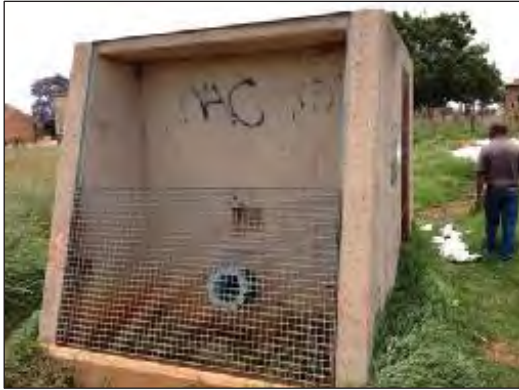
Ekangala-Enkeldoornoog Aqueduct facility
