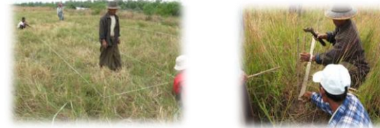
Measuring and Lining Planned Pond Area
