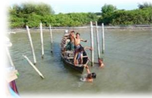
Piling posts and connecting each post by rope.
