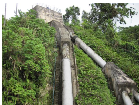
Photo 2: Steel Pipe Installed (Left)
