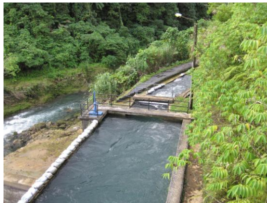
Photo 1: Current Condition of the Intake Water Canal
