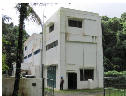
Photo 3: Hydroelectric Power Station Overview
