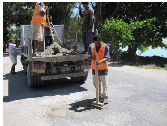
Photo 3: Road Maintenance Work (Non-Project Section)
