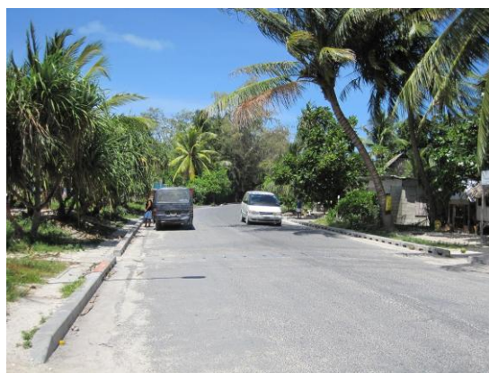
Road Section Improved in the Project
