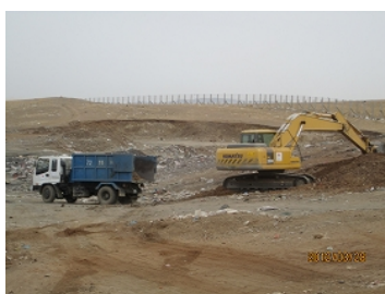
Heavy machineries provided by the project working at NEDS
