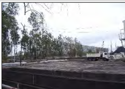
Windbreak Fence installed in the Project
