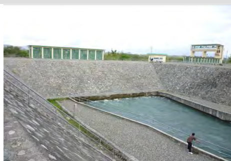
Super Diversion Canal of CMIPP-IC
