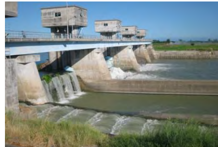
Pampanga Diversion Dam
