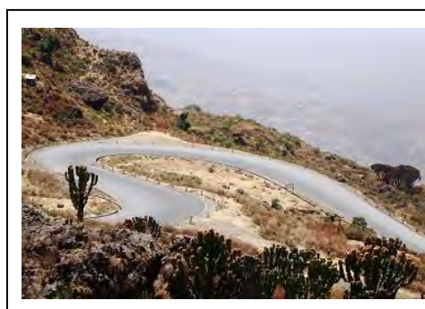
(Abay Gorge and Rehabilitated Road)
