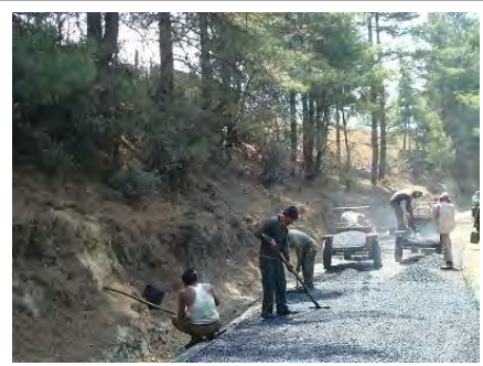
Road construction by NFW
