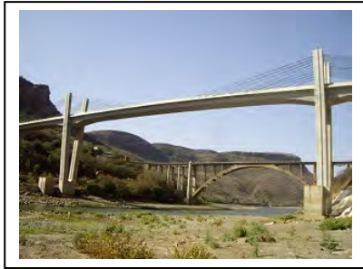
(Abay Bridge (New/front, Old/back))
