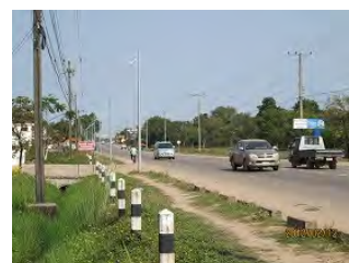
Section that was repaired several times
