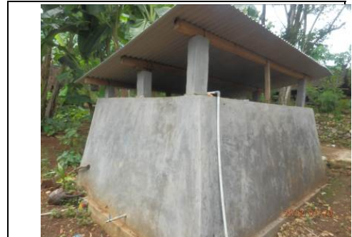
Photo: Common reservoir tank used by the inhabitants. Water supplied from PDAM is stored through pipes and rainwater and tap water are mixed there and used.
