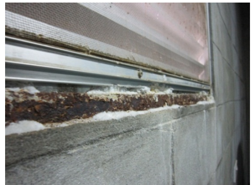
Photo: A window sash on which salt is deposited because wind brings salt
