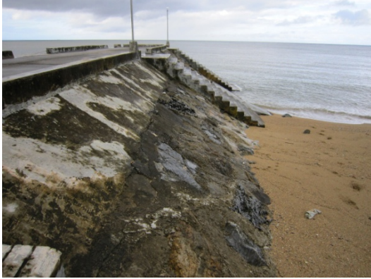
Photo: Repaired part of causeway (Alegria port)
