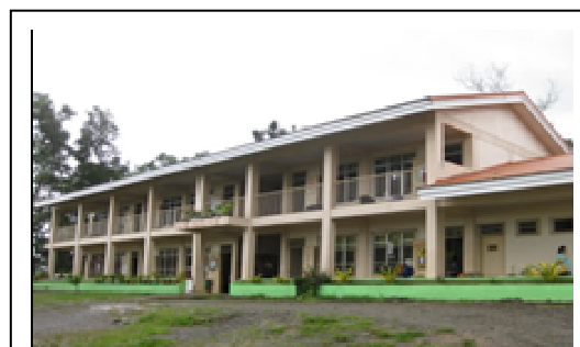
Figure 2. School Building Supported by the Project
