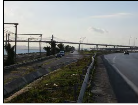
Rades-La Gourette Bridge and Ramps
