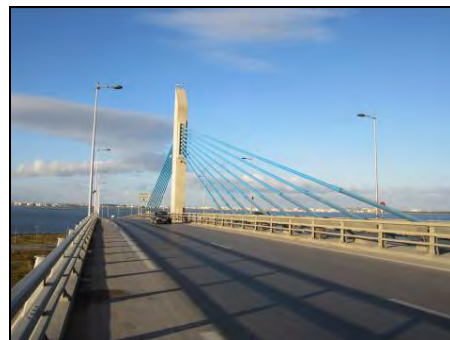
Rades - La Goulette Bridge
