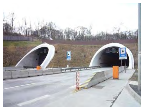
The Tunnel Constructed by the Project
