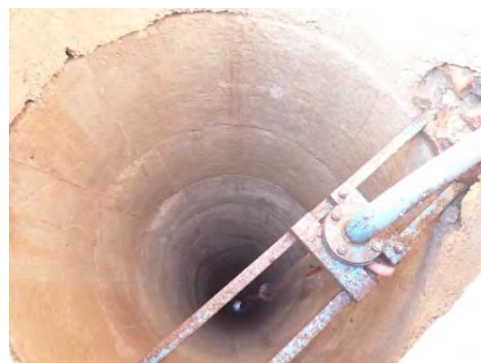
Well excavated in MR-P15
