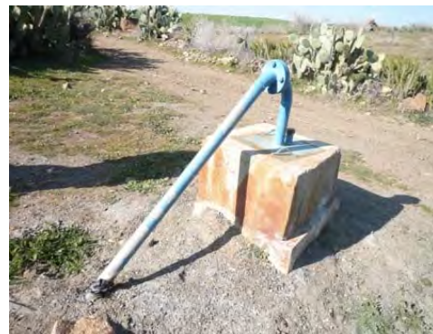
Borehole in Khouribga (MR-P15)
