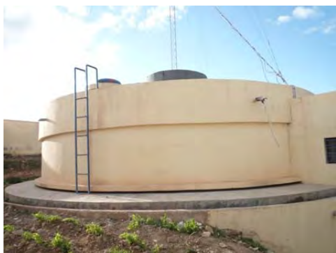
Reservoir constructed in MR-P14
