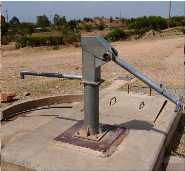
A Manual Standpipe Near the Outlet Channel
