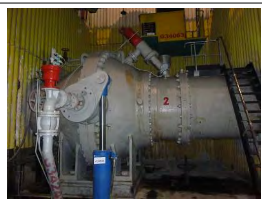
Renewed Water Valve of Khrami II Power Station
