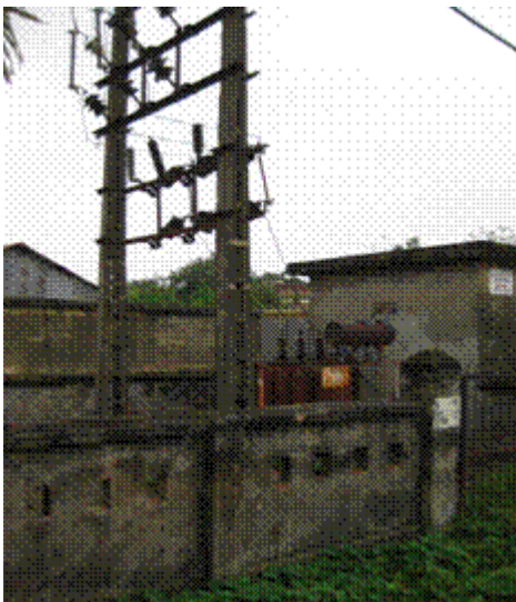
(Outdated substation in a village dating to the 70's)
