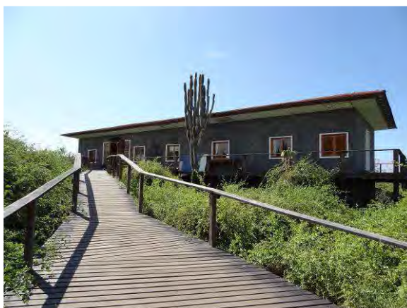
Newly constructed Project Office (currently used as the PNG Office)
