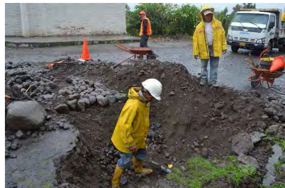
Works for water leakage prevention
