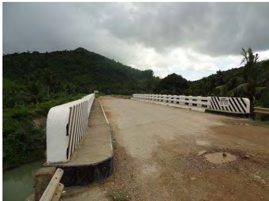
The upgraded bridge (Taytay-El Nido)
