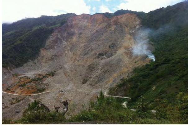
Fig. 2 Current State of the Major Landslide Site at Los Chorros on RN-7W
