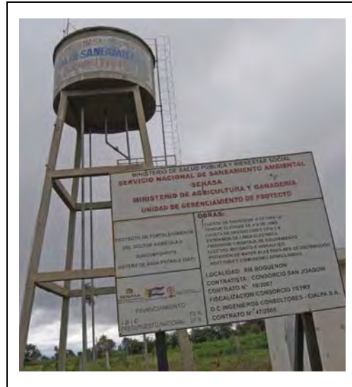
(A water supply tank installed in the community)
