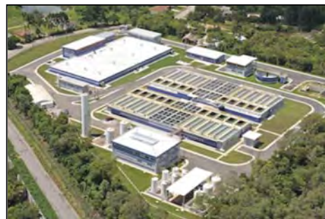
Miringuava Water Treatment Plant
