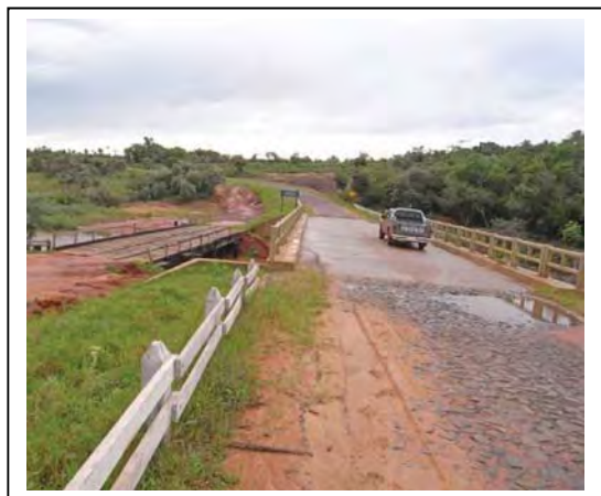
(Left: Old wooden bridge, Right: New concrete bridge)
