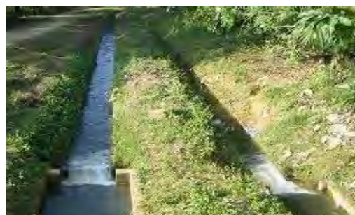
Dual Canal System: The left canal is for paddy and the right canal is for OFC
