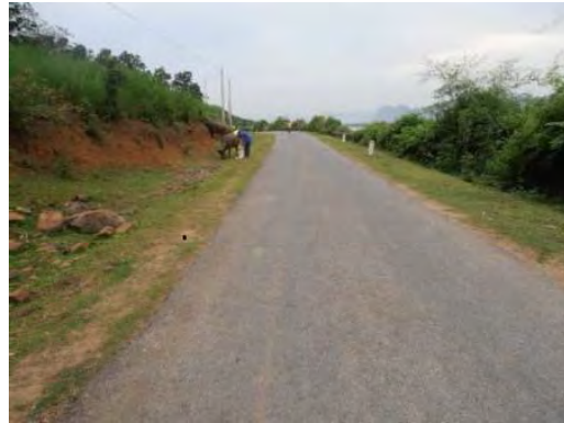
District road constructed by the project
