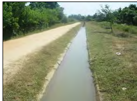
Rehabilitated Irrigation Canal
