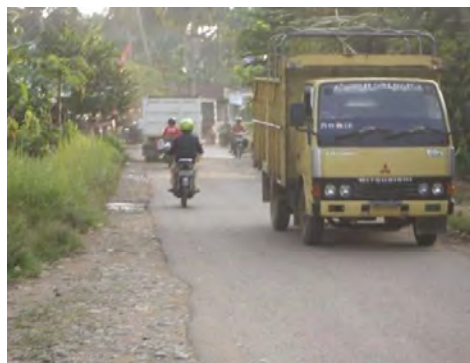
Former Inspection Road Regional Major Transport Media after Project
