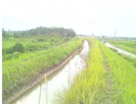
Secondary Canal Arid Soil Turned Watery
