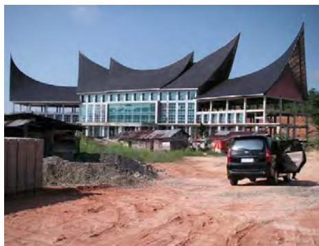
Regional Hospital under Construction
