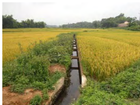
Irrigation canal constructed by the project and grown rice
