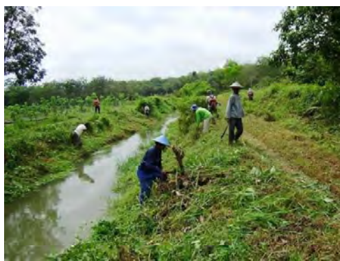
Canal Maintenance Work by Farmers
