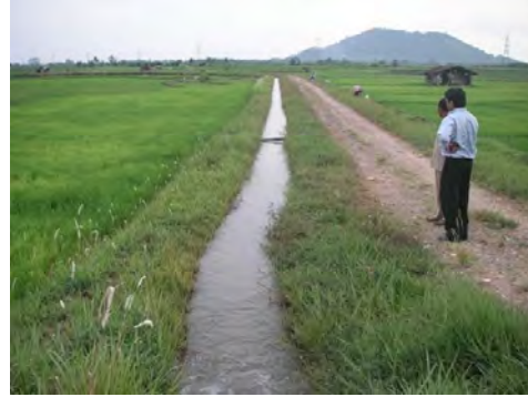
Tertiary Canal Extending to Farm Fields
