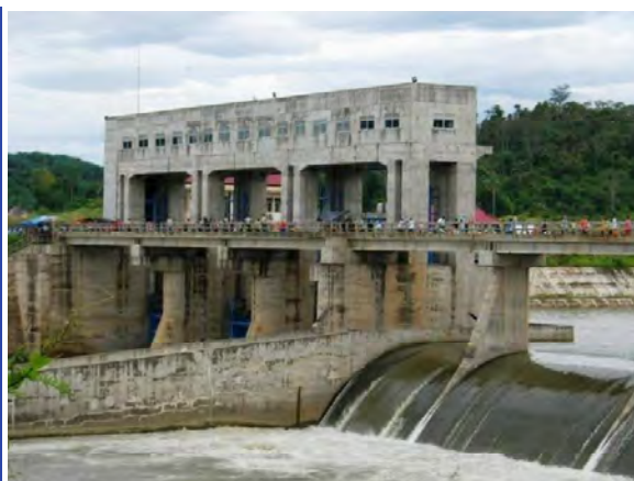
Completed Batang Hari Weir
