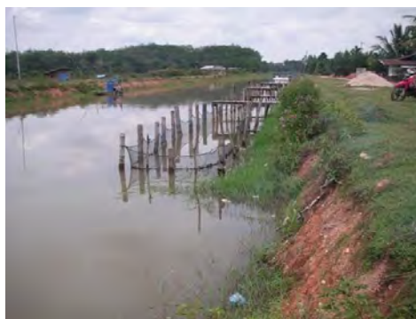
Installed Aquaculture Cage on Primary Canal
