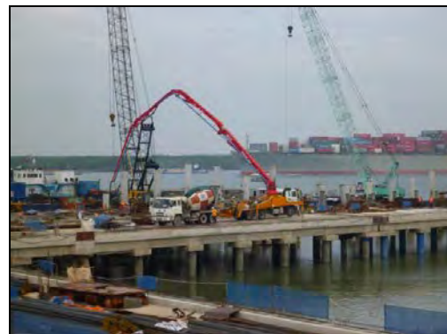
Cai Mep Terminal under construction
