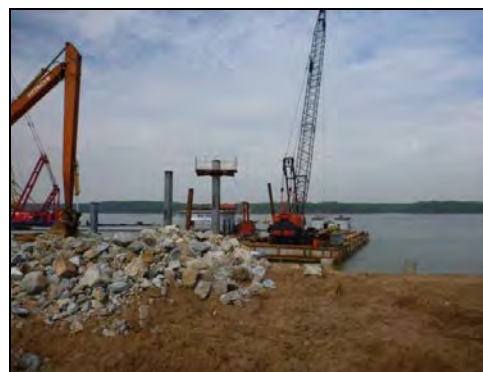
Photo 1: Thi Vai Terminal under construction
