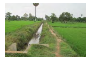
Tertiary canal rehabilitated by Cambodia side
