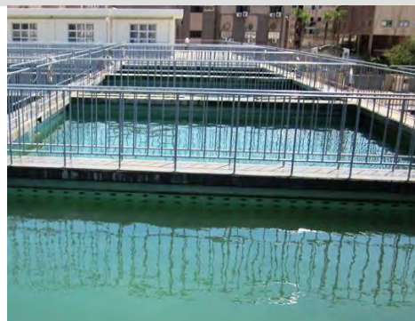
Coagulation Sedimentation Basins
