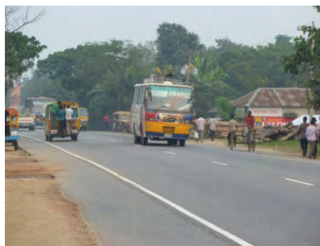
Road Developed by the Project
