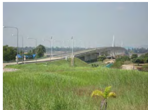
Second Mekong International Bridge (taken from Lao side)
