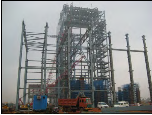
Construction of the NHPC Vizag Thermal Power Plant (As of December 2011)
