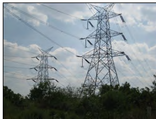
400kV Transmission Line constructed by the Project
