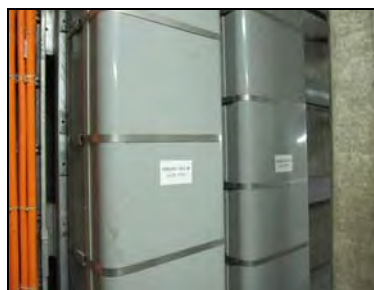
Transmission Line Trough
