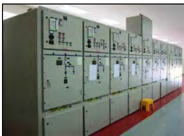
Switchgear in Chiang Dao S/S
