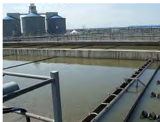
No.4 Wastewater Treatment Plant
