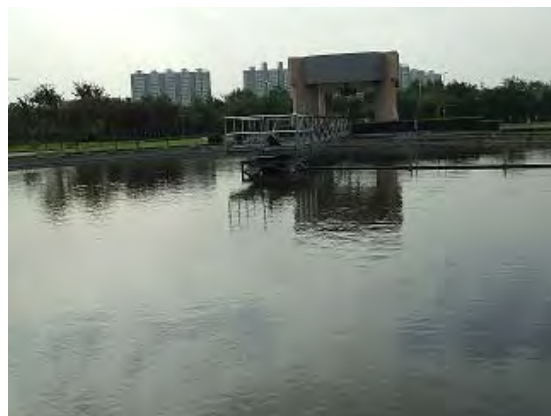
No. 3 Wastewater Treatment Plant
