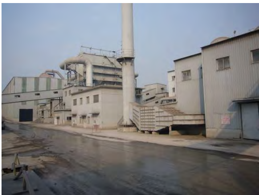
Steel dregs treatment plant
