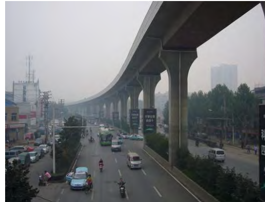
Tracks on viaduct section (Jinghan Avenue)
