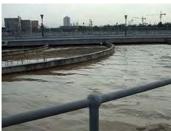
No.3 Wastewater Treatment Plant (Orbal oxidation ditch)
