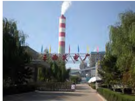
Wangqu Thermal Power Plant
