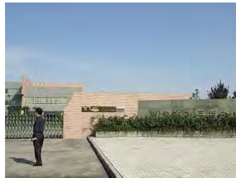
Xi'an No.3 Wastewater Treatment Plant
