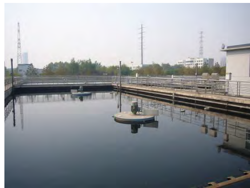
Sewage Treatment Plant
