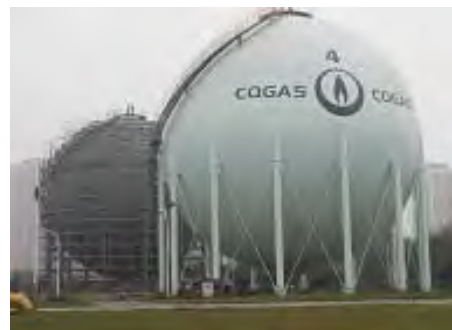
Toutong Natural Gas Station
