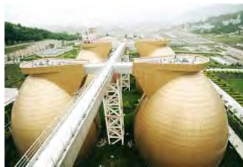
Jiguanshi Wastewater Treatment Plant Digestion Tank
