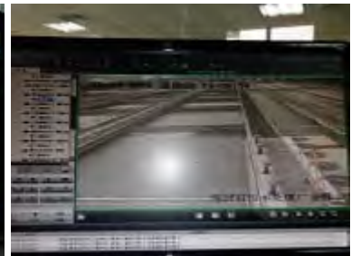
Real-time picture of camera at Jiguanshi Wastewater Treatment Plant
