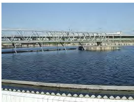
No.4 Wastewater Treatment Plant
