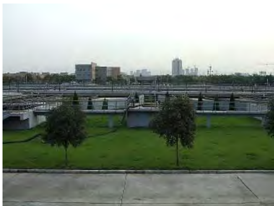
No. 3 Wastewater Treatment Plant
