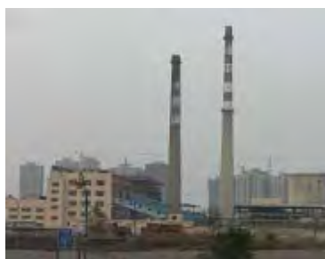
Full view of Yendao Thermal Power Station
